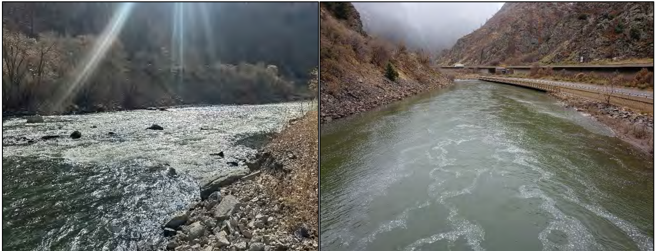
Figure 5. (Left) Looking downstream from the right bank at the rapid in the middle of the survey area. (Right) Aerial oblique drone photo looking downstream from near the upstream end of the survey area. The riprap and concrete nature of the banks can be seen.
