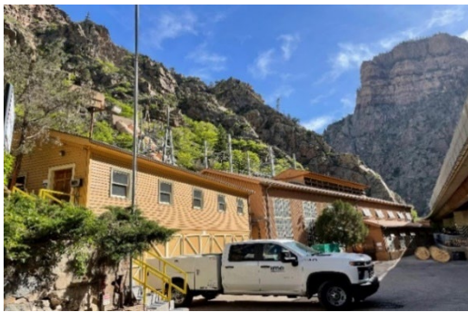
Figure 1: Shoshone Power Plant
