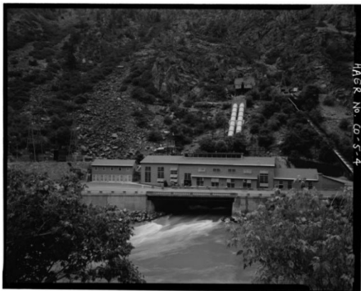
Figure 12: Shoshone Power Plant, Library of Congress
